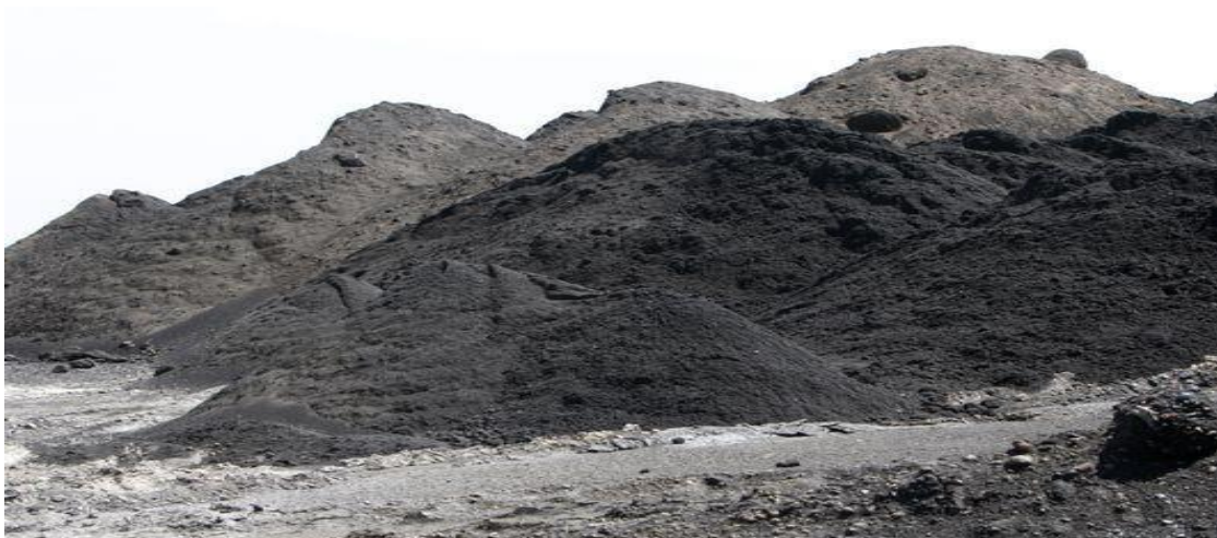
Fig 1: Fly ash disposal in landfills (dry method).
